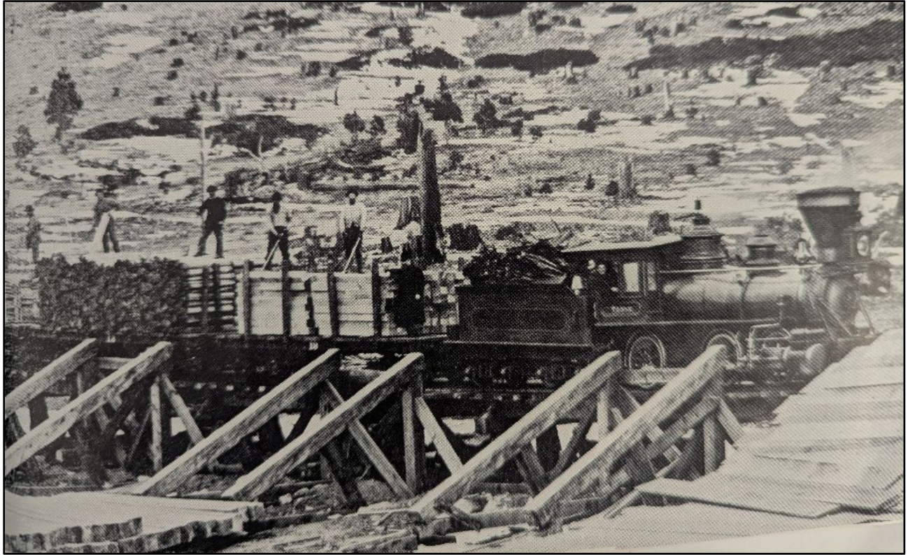
At Spooner Summit, milled lumber was unloaded from of C&TL&F trains and into a V-shaped flume, which floated the lumber 11 miles from the summit to Carson City. In this photo the locomotive Tahoe heads the train at the unloading facility located just east of the summit tunnel for the railroad.
